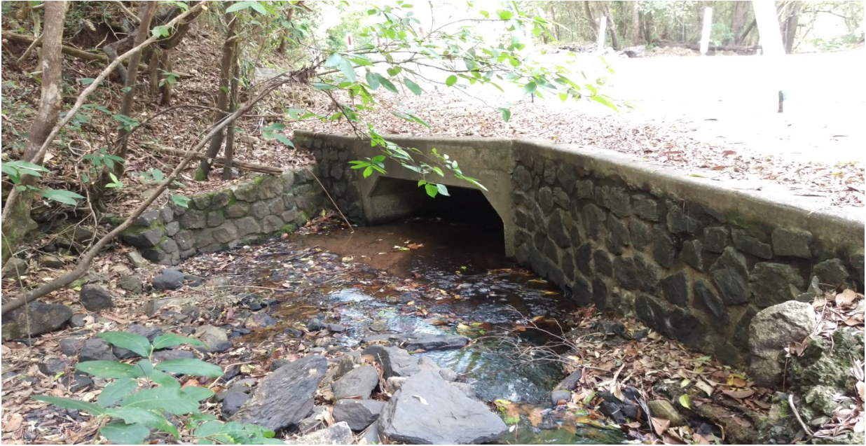
Upstream of Gold Creek Road #7
