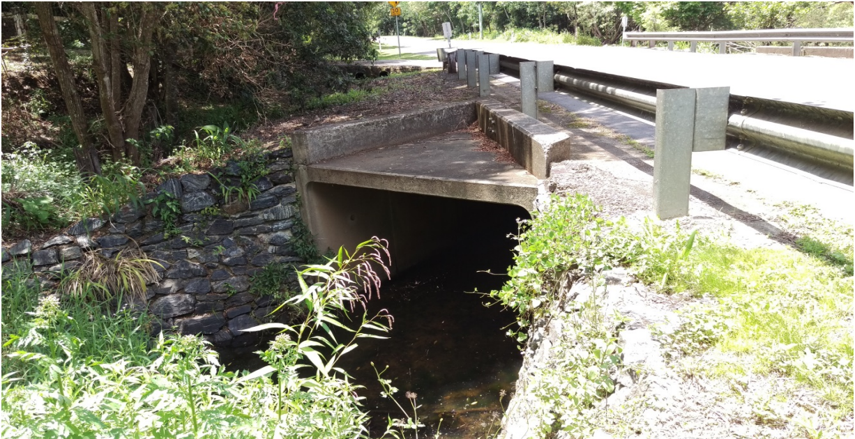
Upstream of Gold Creek Road #3
