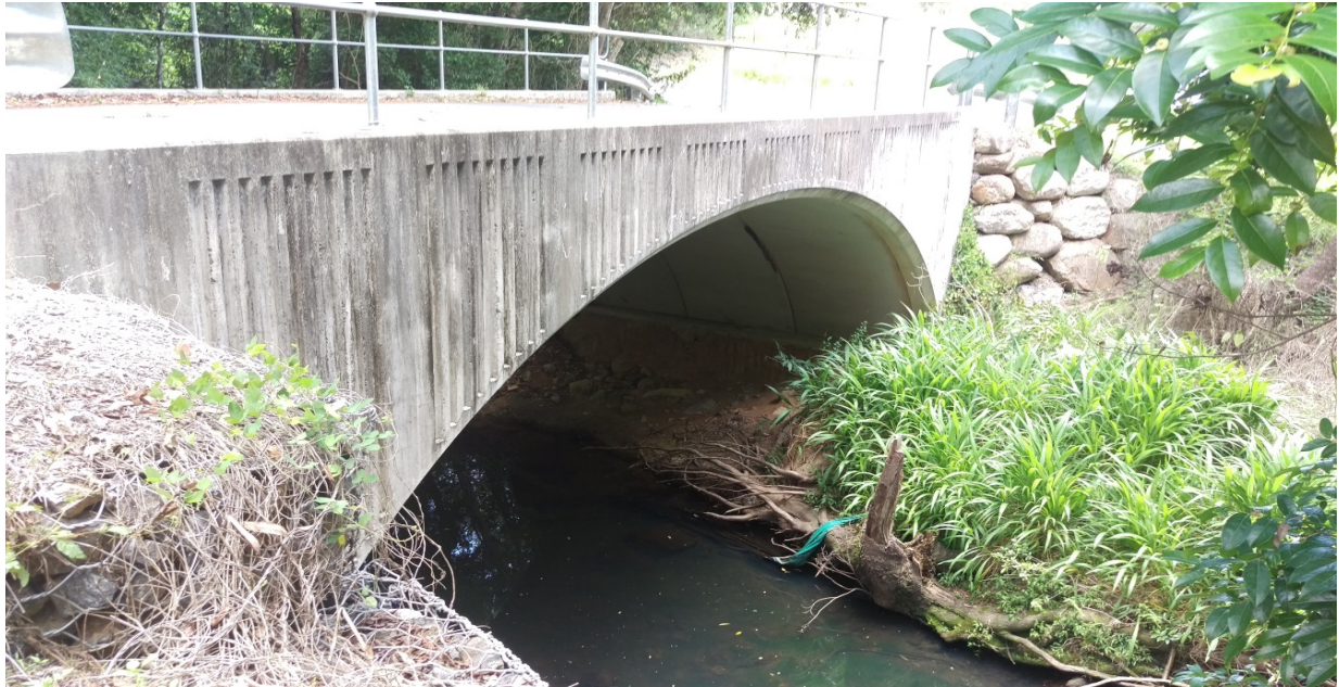
Upstream of 272 Gold Creek Road
