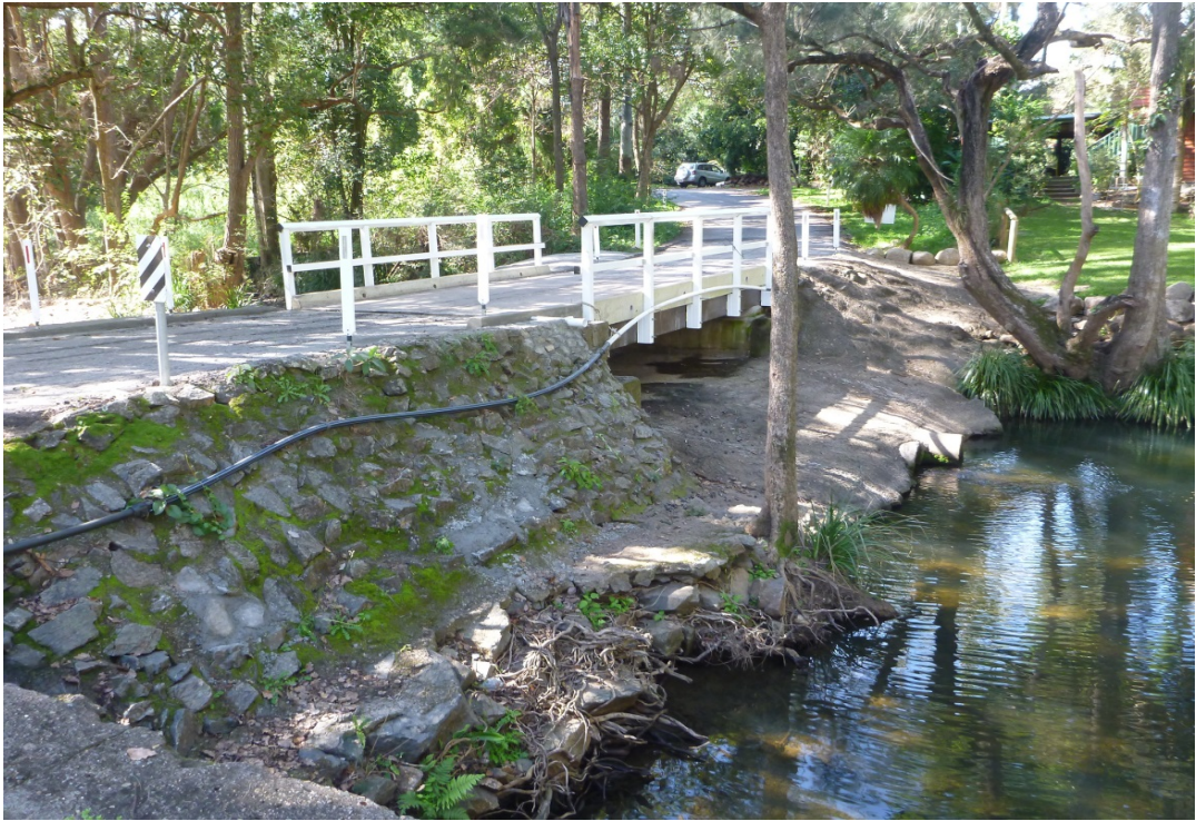
Downstream of Bundaleer Street
