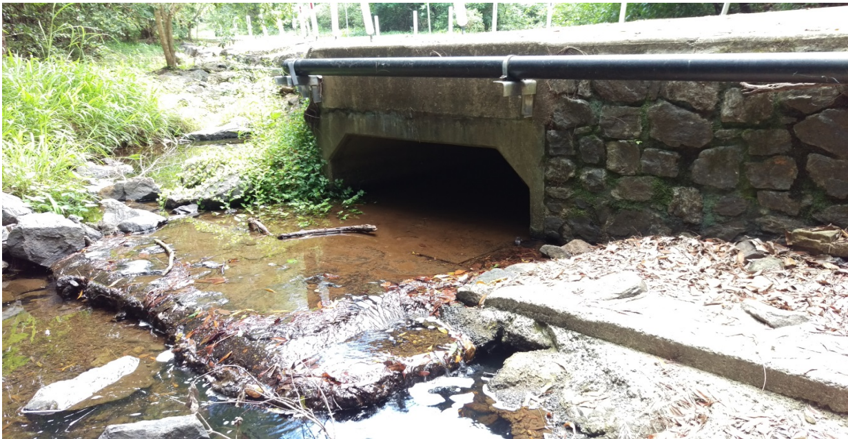
Downstream of Gold Creek Road #7
