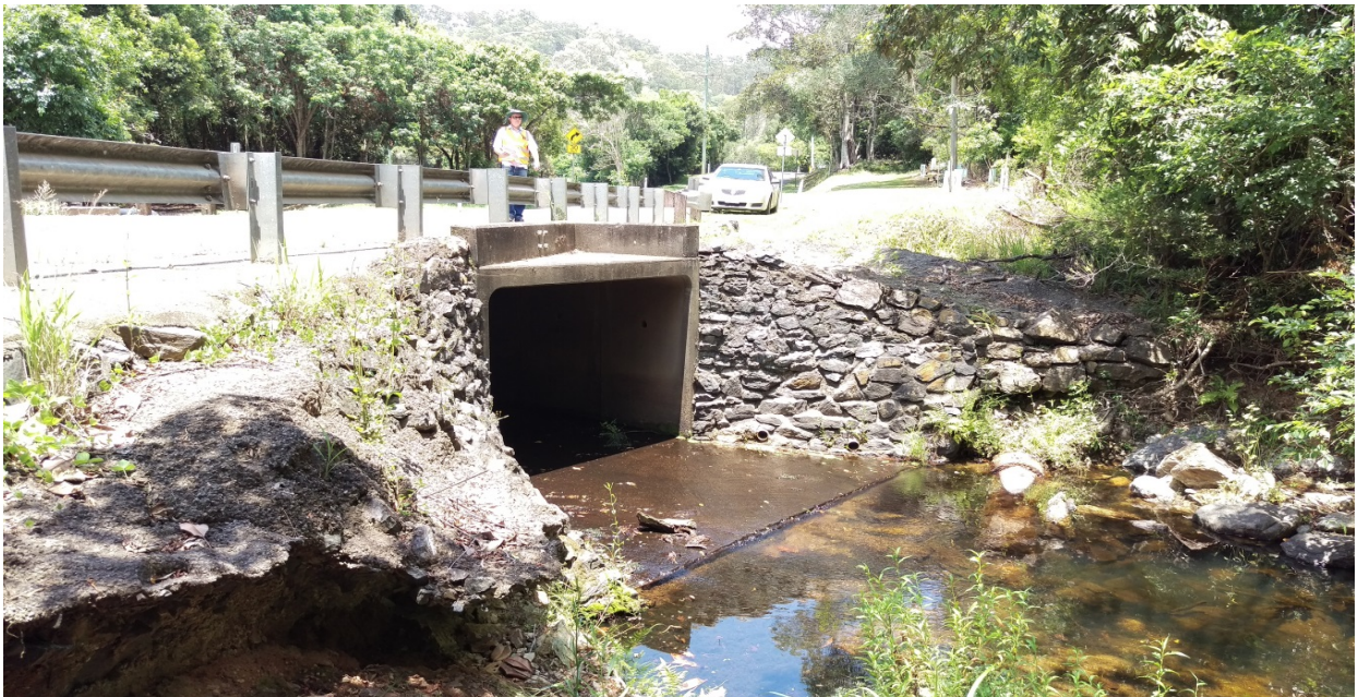
Downstream of Gold Creek Road #2
