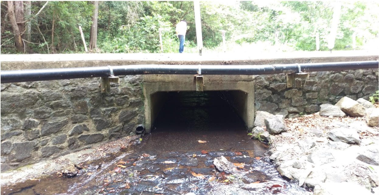
Downstream of Gold Creek Road #8
