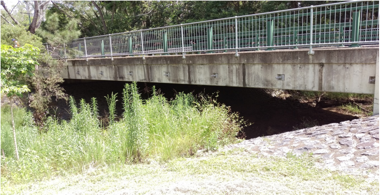
Upstream of Brookfield Road (Gap Creek)
