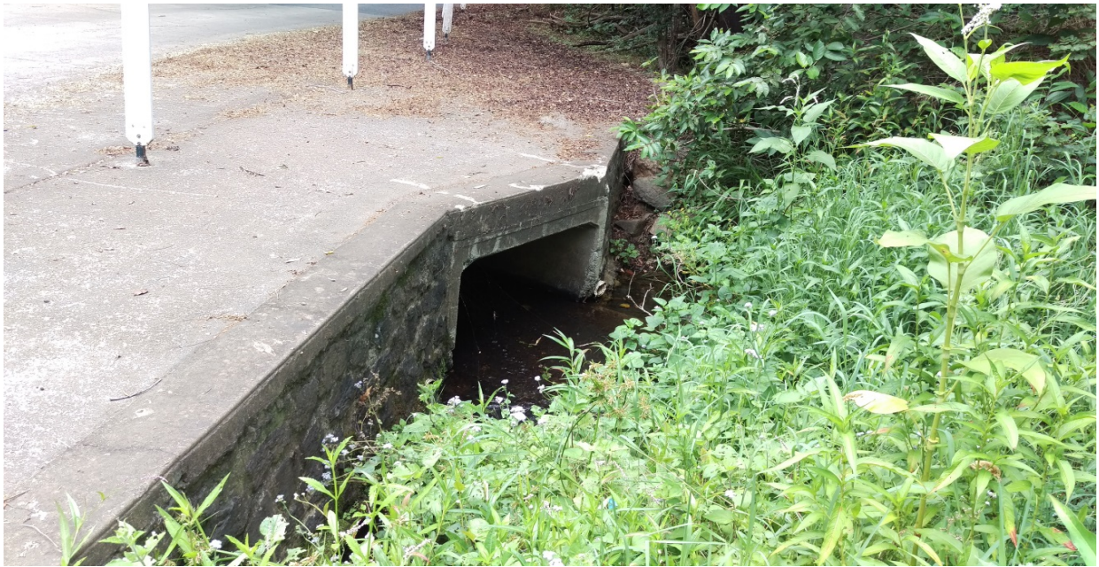
Upstream of Gold Creek Road #8
