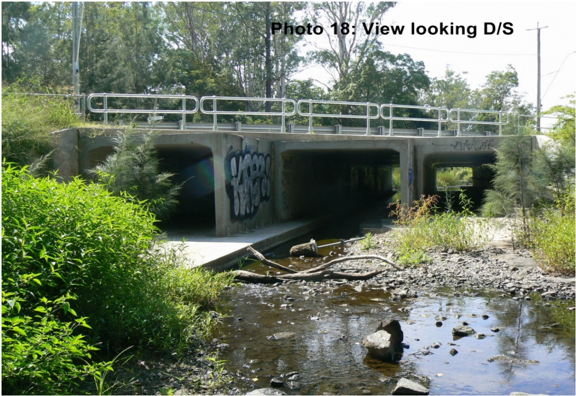
Upstream of Rafting Ground Road Culvert 1
