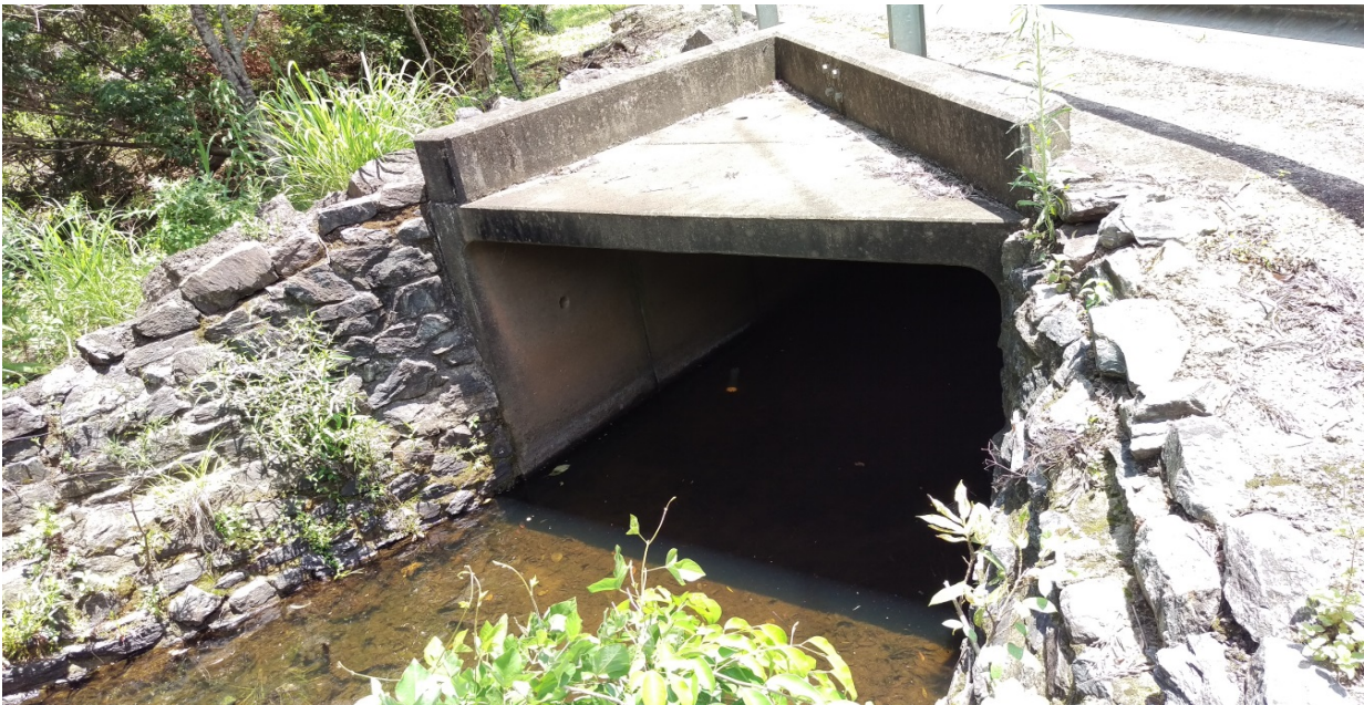
Downstream of Gold Creek Road #3
