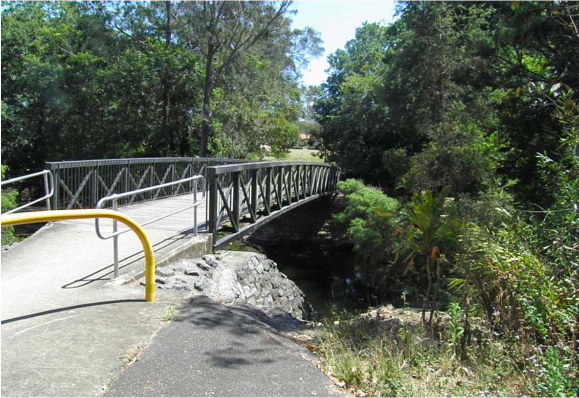
Upstream of Branton Street Footbridge
