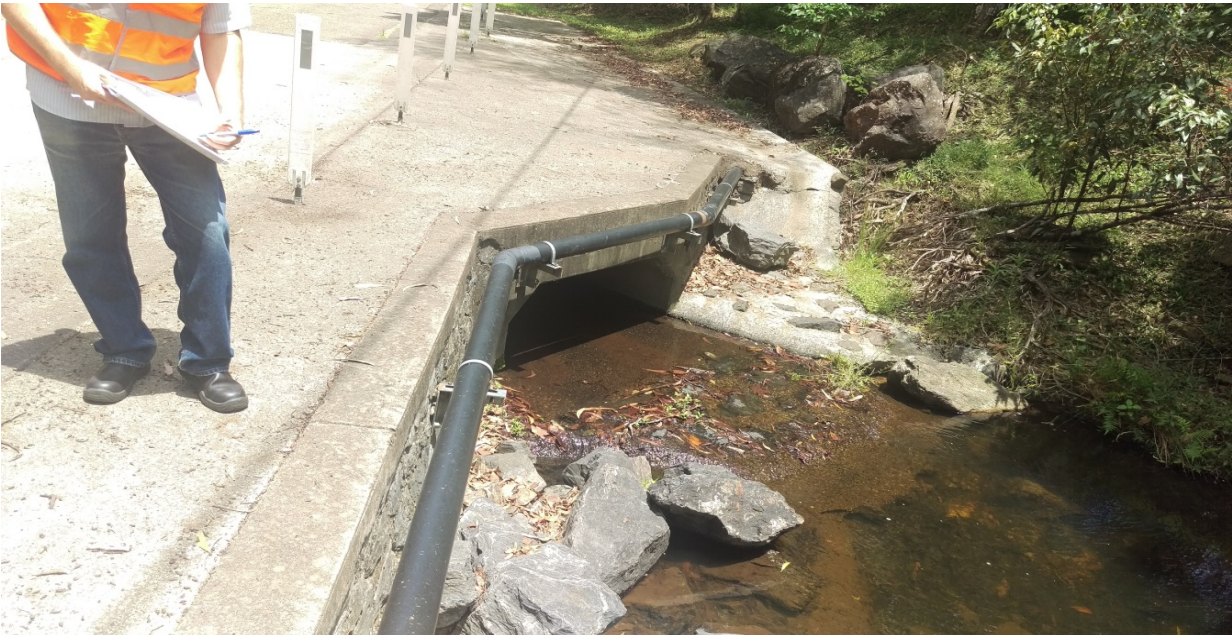
Downstream of Gold Creek Road #6
