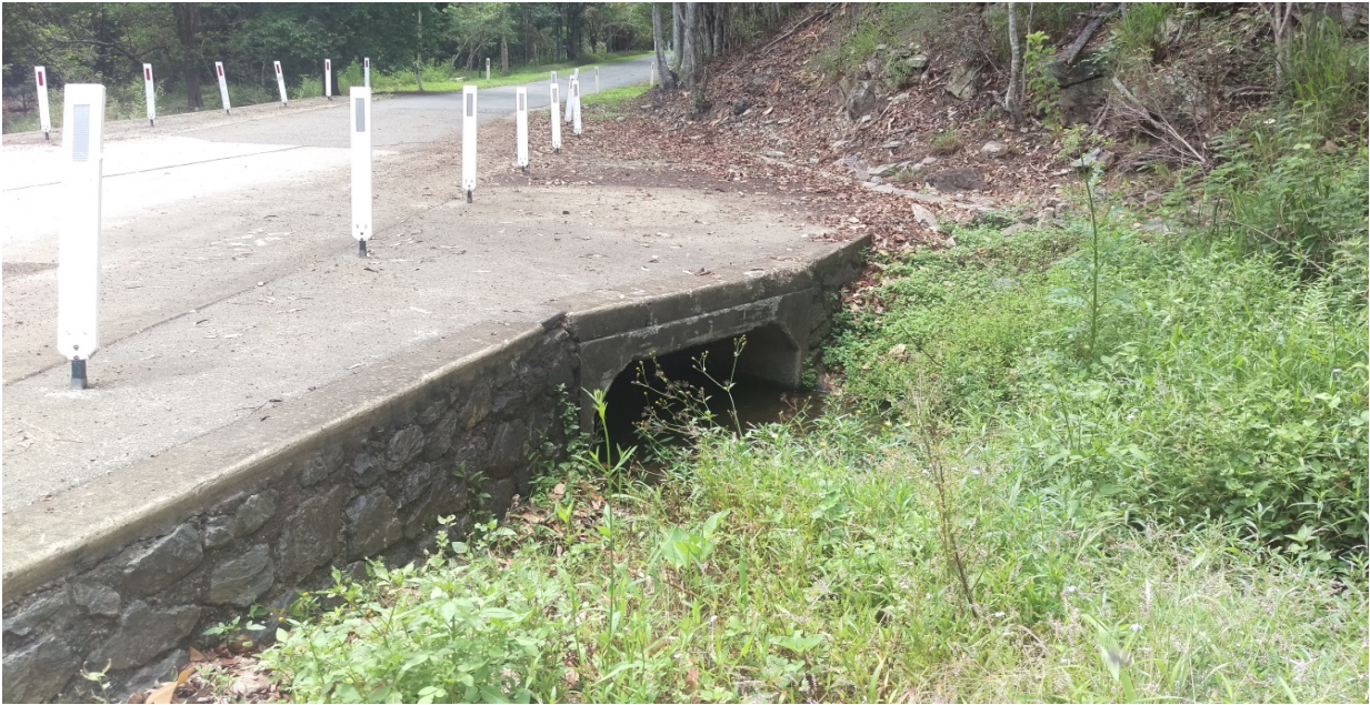
Upstream of Gold Creek Road #6
