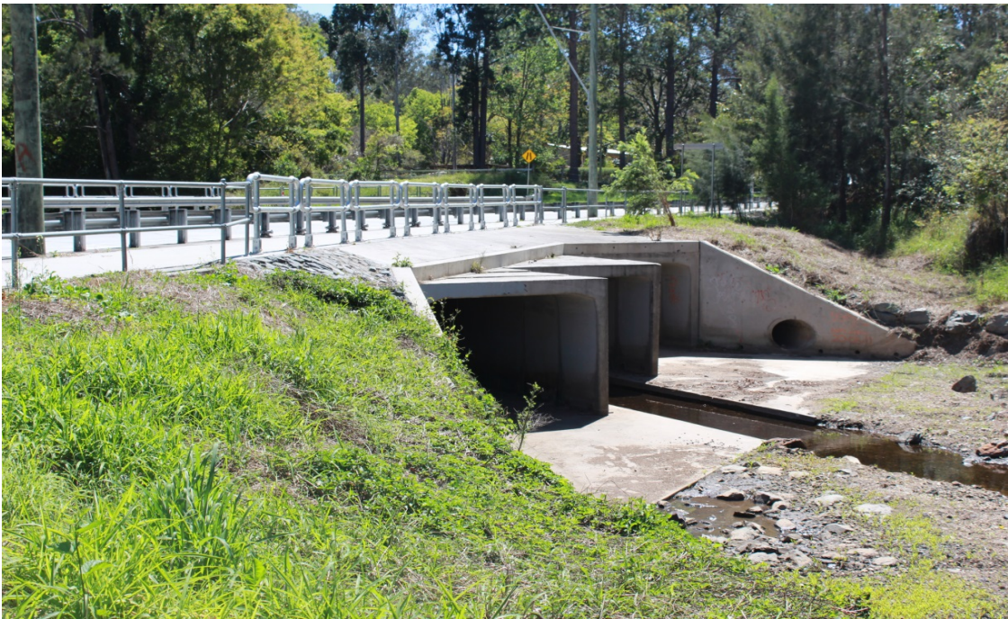
Downstream of Rafting Ground Road Culvert 1
