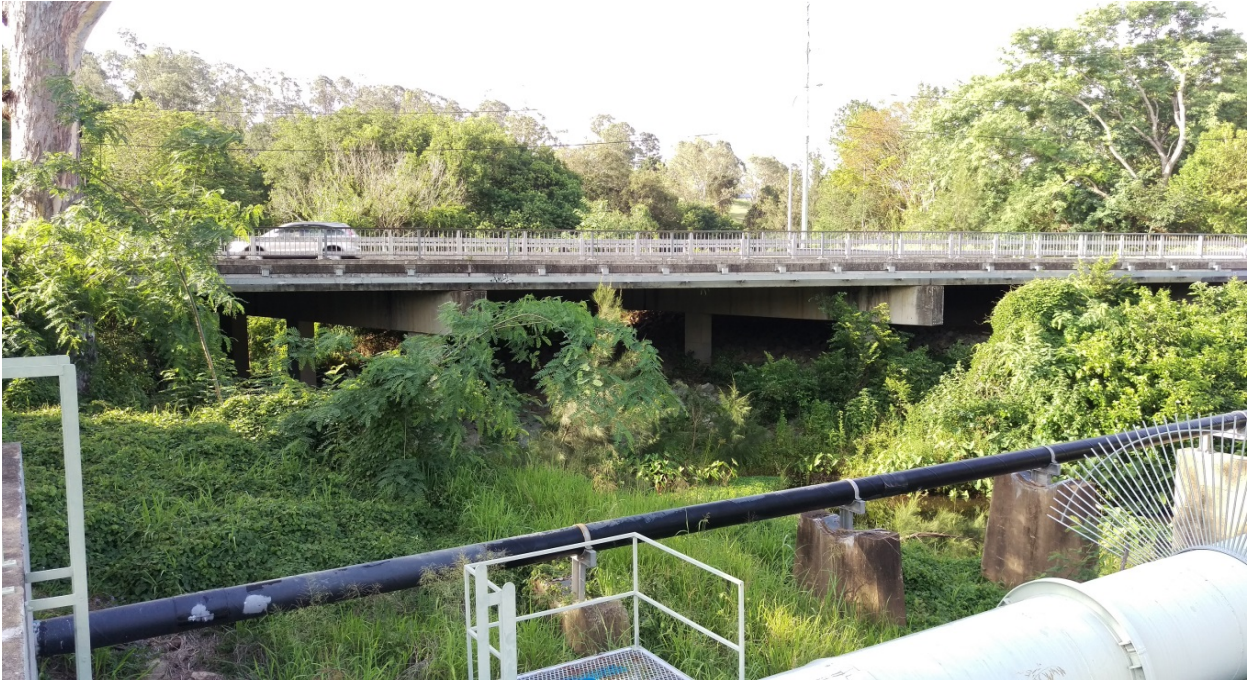
Downstream of Moggill Road Bridge
