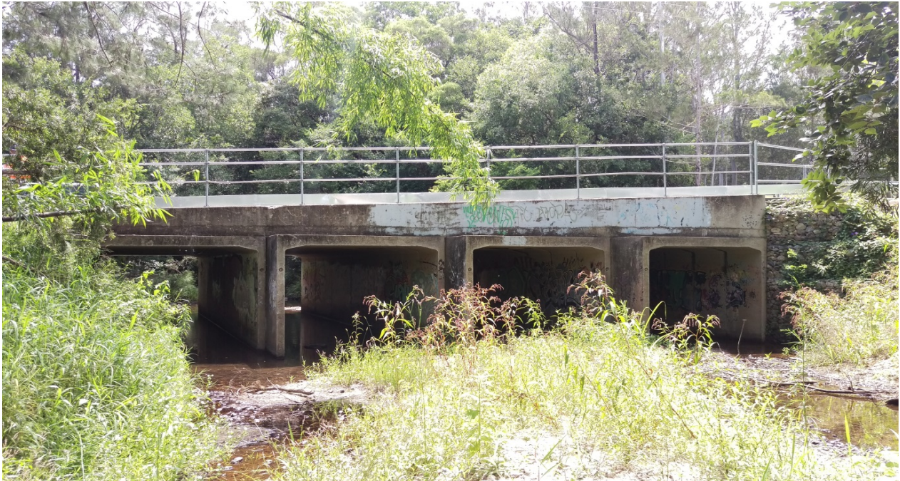
Upstream of Rafting Ground Road 2 Culverts
