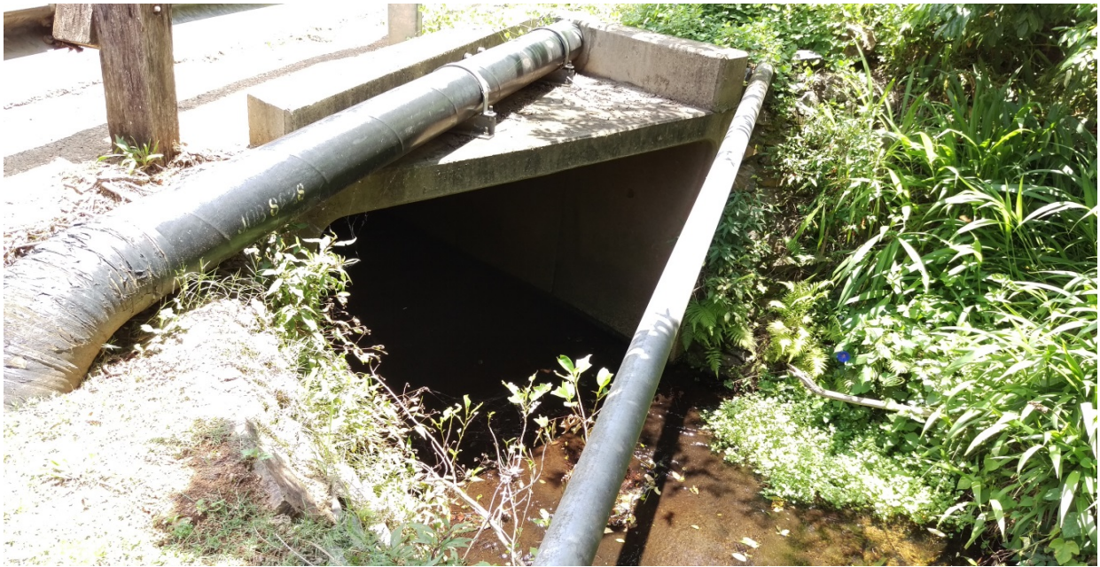
Upstream of Gold Creek Road #2
