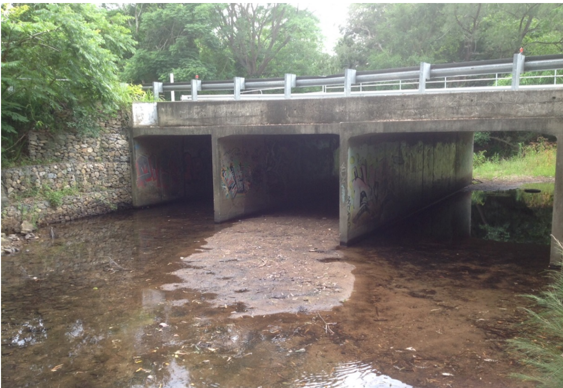
Downstream of Rafting Ground Road 2 Culverts
