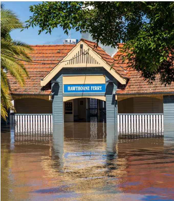
Hawthorne Ferry Terminal
