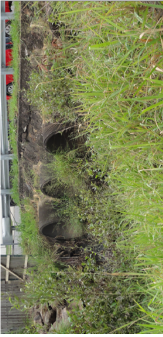
Photo 2 - Outlet Structure (heavy vegetation)
