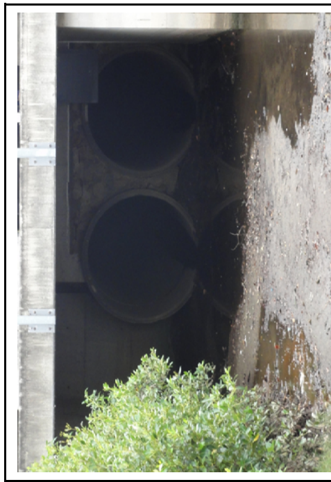
Photo 2 - Outlet Structure (Right bank culverts)
