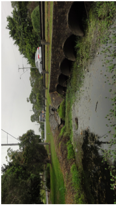
Photo 1 - Culvert inlet structure -sedimentation and water clogging
