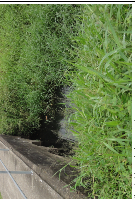
Photo 3 - Culvert outlet - heavy vegetation
