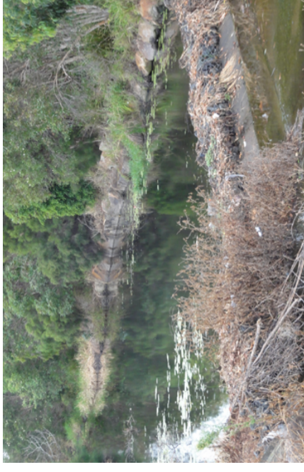
Photo 2 - Upstream weir pool
