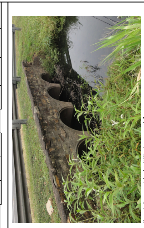
Photo 3 - Culvert outlet - heavy vegetation
