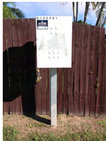
TYPICAL MOUNTED SWITCHBOARD
