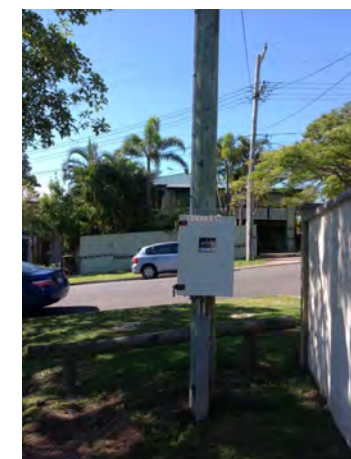
TYPICAL MOUNTED SWITCHBOARD
